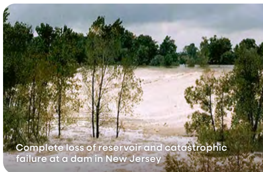
Overtopping can fail an earthen dam
