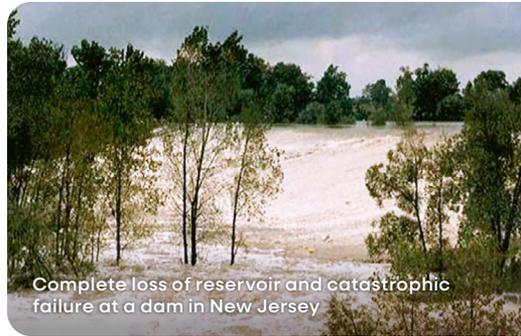
Complete loss of reservoir and catastrophic failure at a dam in New Jersey
