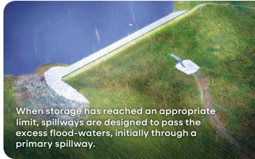
When storage has reached an appropriate limit, spillways are designed to pass the excess flood-waters, initially through a primary spillway.
