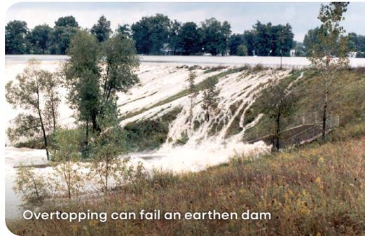
Overtopping can fail an earthen dam
