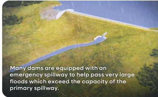
Many dams are equipped with an emergency spillway to help pass very large floods which exceed the capacity of the primary spillway.
