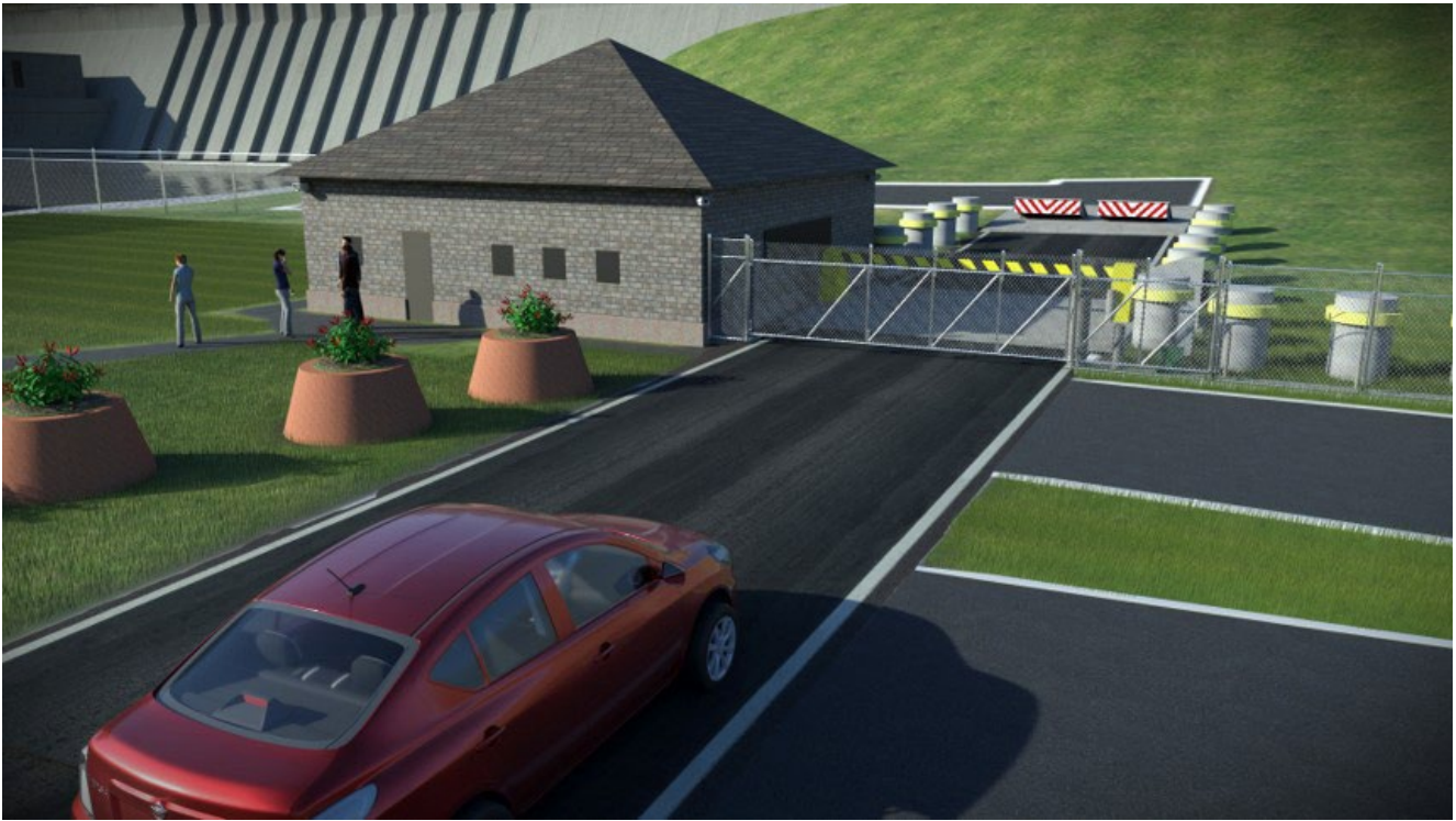
Figure C4. Inset 2 from Figure C2 (Entry Control Point with Active Barriers) Source: U.S. Army Corps of Engineers
