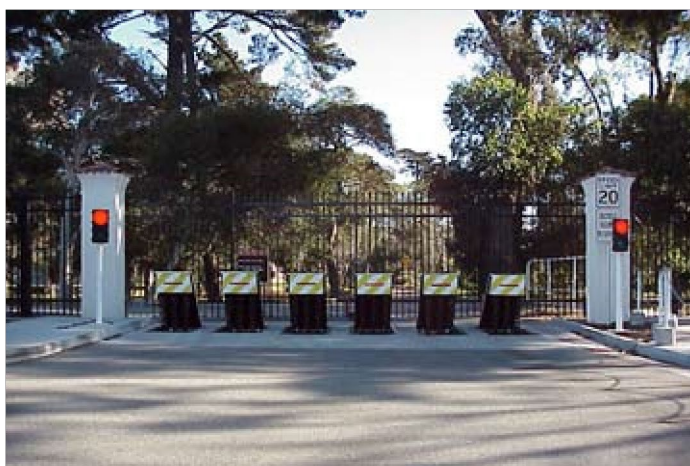
Figure 2. Use of Active and Passive Barriers
